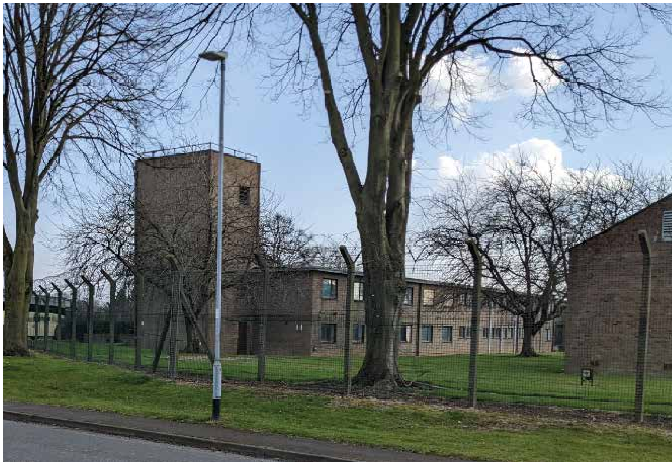
View of the site from Manton Road.
